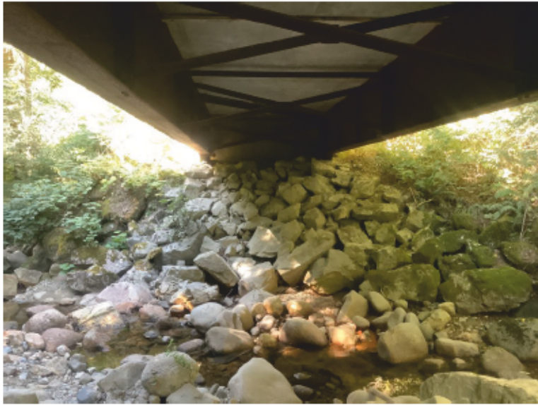
Right Bank Abutment when facing downstream
