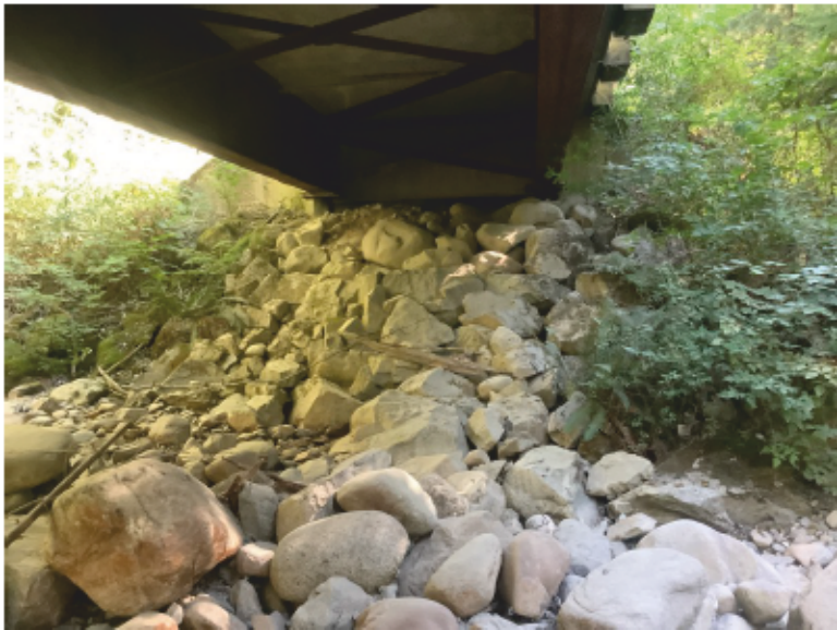
Left Bank Abutment when facing downstream
